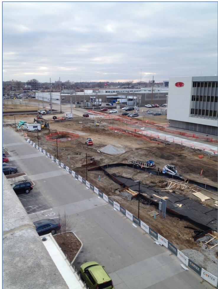
View of the Commons construction from the roof of @4240
